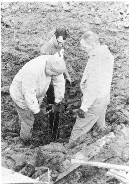
Iron probing rods are used by workers to detect objects in the soft mixture of clay and wet soil.
