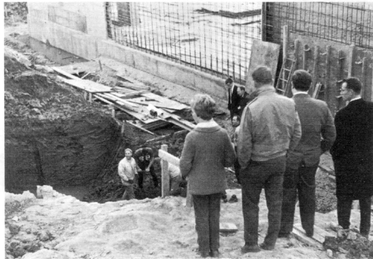
Interested onlookers view the digging operations from a dry vantage point.
